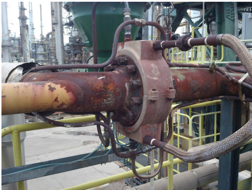
Figure 2 – Tracing and Insulation for sulfur pit vent gas
